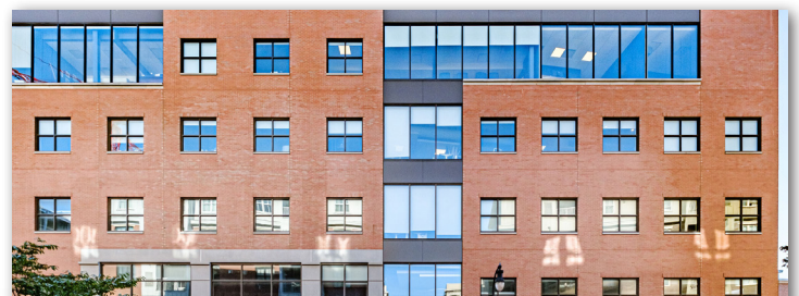
16 Middle Street, Portland
