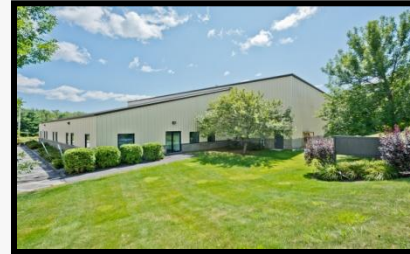
921 Riverside Street, Portland 25,000 SF
